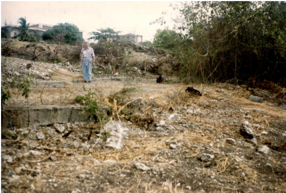
Figure 3 Flat step of the first reversal at the top of Gibbons hill. Street construction had begun on the flat of the step. E.G. Johnson assisted.
