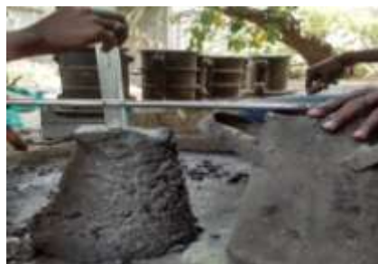
Fig. 4 Slump Test on a Typical Concrete Mix
