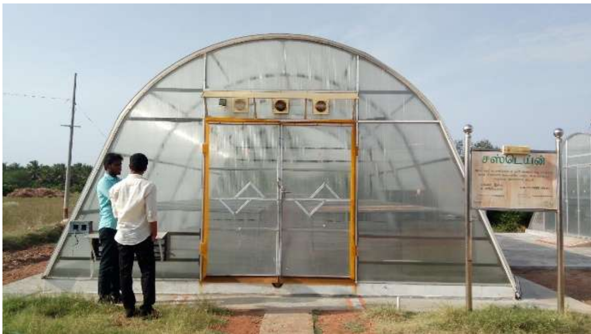
Figure 2 Front end view of the Solar Greenhouse dryer
