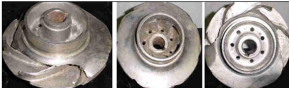
Fig.8 – Corrosion-erosion of a stainless steel rotor
