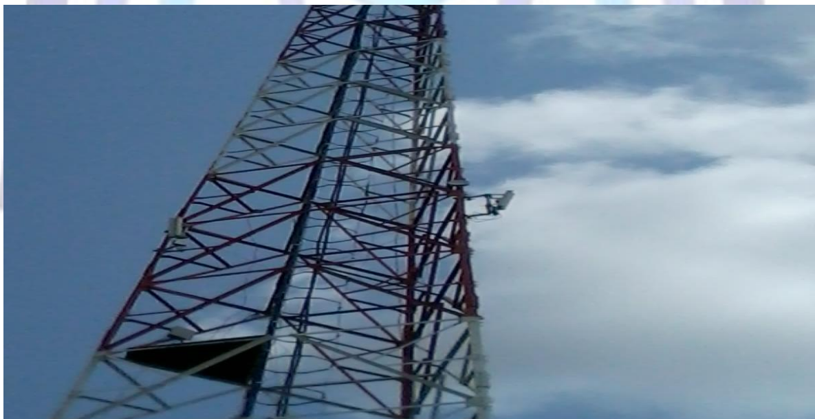
Figure 7: Antenna mast with Tranzeo and wavion radios (experimental testbed)
